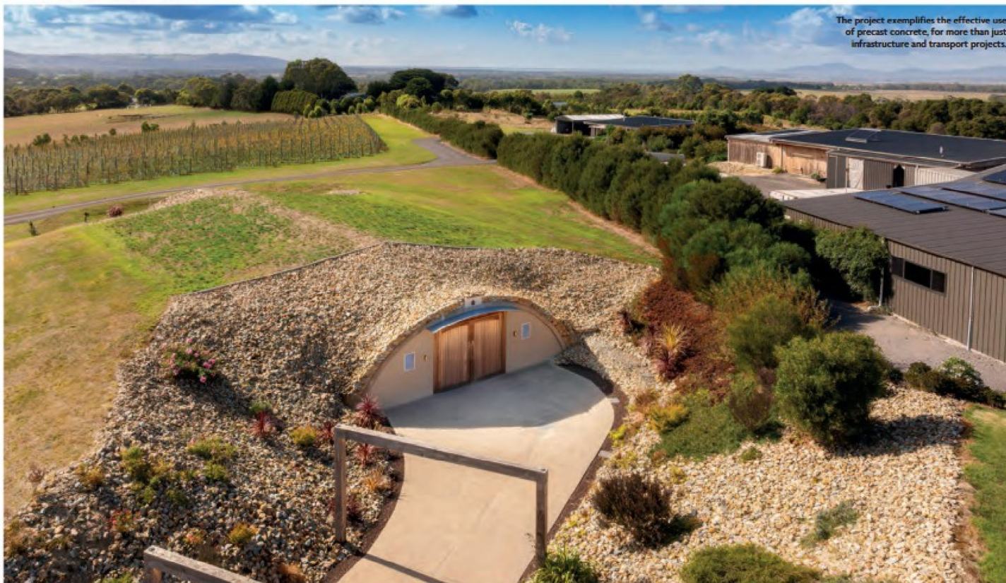
The arch system has been delivered by using precast to create a subsurface storage facility.
