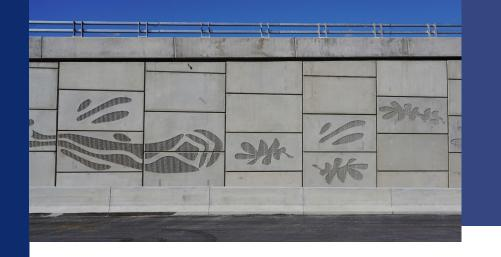
According to the Geoquest's Managing Director in Australia Riccardo Musella, the walls provide not only structural integrity, but also flexibility in design, thanks to custom-made form liners that allow for unique urban patterns on the panels.
