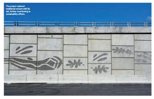
integrity, but also flexibility in design, thanks to custom-made form liners that allow for unique urban patterns on the panels.
