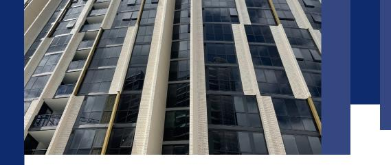
Among the standout features of the precast elements are 562 wall panels and 605 spandrel panels, which have been directly connected to the structural slab for structural stability and durability, both during construction and throughout the building's life.
