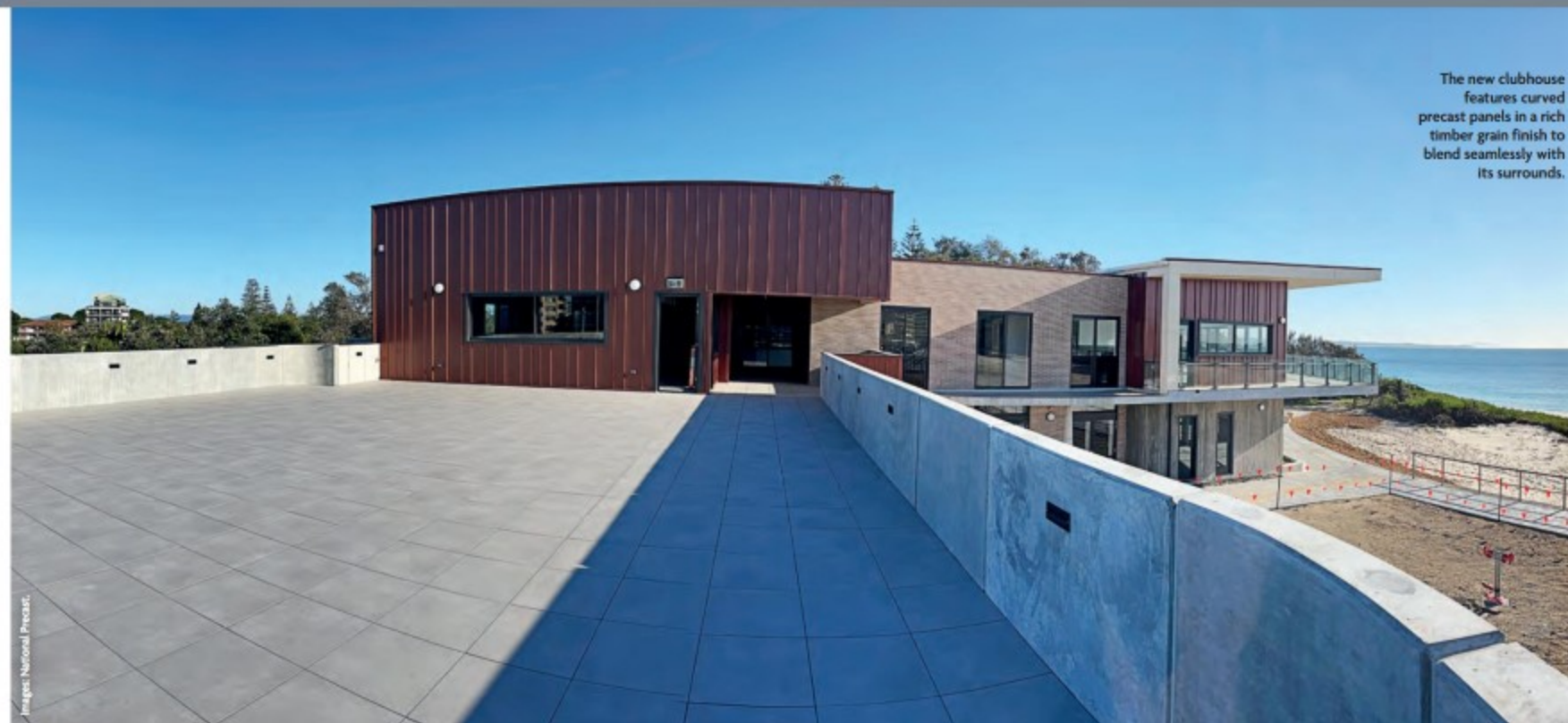
Using precast panels allowed for earlier completion.
