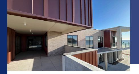
Additionally, the balcony panels are equipped with pre-installed electric lights and power conduits. Being installed in the factory before delivery, offered time saving benefits on site and ensured the high quality that was demanded to ensure both safety and functionality.
