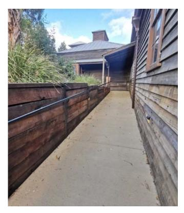
According to Sunset Sleepers Director Miguel Donnenfeld, 800 customdesigned reinforced concrete sleepers were custom-manufactured, tailored to specific engineering requirements. R6 rebar was specified in the project drawings, to enhance durability and prevent shear failure. By distributing stresses more evenly throughout the sleepers, the reinforcement would also control shrinkage and potential cracking during construction.
