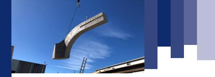
Over 300 grooved wall panels – which included numerous curved panels and which measured between 3 and 31 square metres, were manufactured for the East façade. 135 arched and rectangular columns weighing between 5 and 17 tonne were supplied for the main façade, while 4 square metre grooved soffit panels that were triangular in shape feature on George Street. The panels were manufactured using an off-white oxide.
