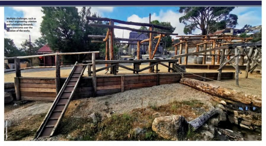
a platform – which required additional retaining walls – to provide wheelchair access to a new all-ability gold panning area.
