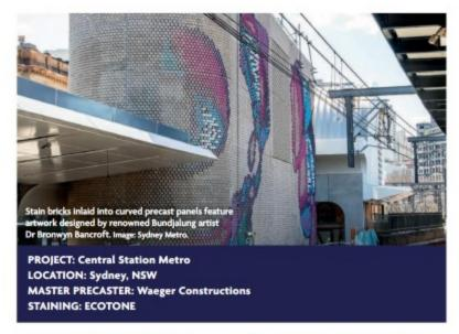
revolution. In this case, the inlaid bricks have been stained, but in many other projects, the precast itself is stained – with or without using form liners to create pattern," says Bachmann. "Traditionally used most commonly to colour correct brickwork and in more recent times cast insitu concrete, staining is now frequently used on precast as well to achieve amazing statements in colour, from translucent, to opaque, to metallic finishes. It is incredibly
