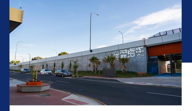
Known as a counterfort retaining wall system, it consists of full-height wall facing units that are secured to a cast-in-place footing. The facing panels – which can easily feature architectural detailing and patterns - are each cast with counterforts on the rear side.
