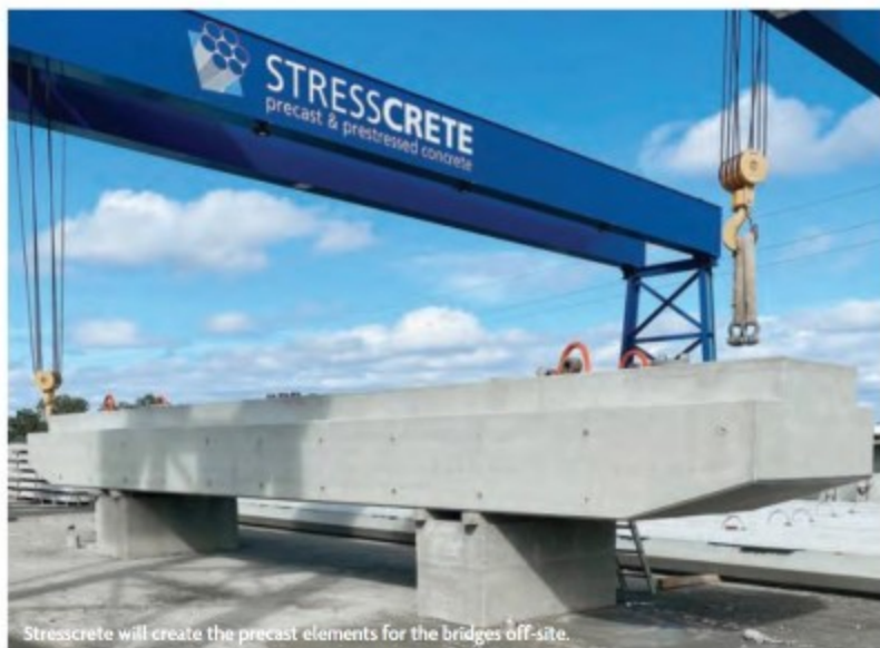
Stresscrete will create the precast elements for the bridges off-site.
