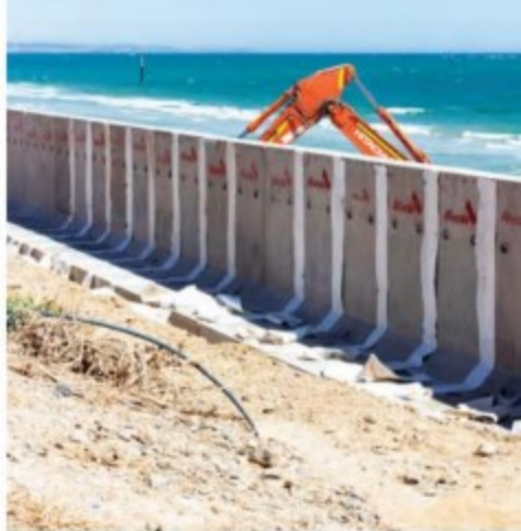
The precast concrete sea wall is designed to protect shoreline erosion.
