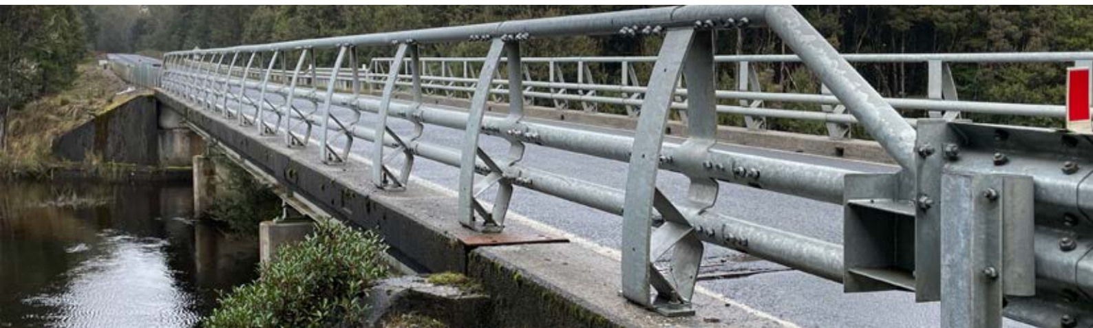
In the two most recent Tasmanian installations, DOLRE barriers replaced old-style steel post and rail barriers with direct connections to concrete kerbs along each of the outer edges of the bridge decks.
