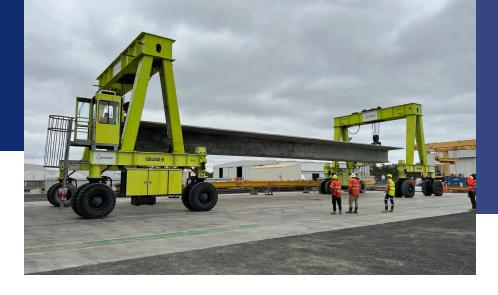
Key to the project are 139 no. precast concrete Teeroff beams, weighing a huge 191 tonne and measuring 41 metres long, 2.2 metres deep by 4.5 metres wide. They have been manufactured for the project by Australian Precast Solutions at their newly built and commissioned factory in Bunbury.
