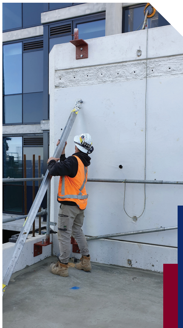
Image 20 – Installation of a brace while the precast element is still supported by the crane
