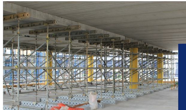
Image 4 – Temporary propping of precast shell beams, (supporting hollowcore flooring) during construction
