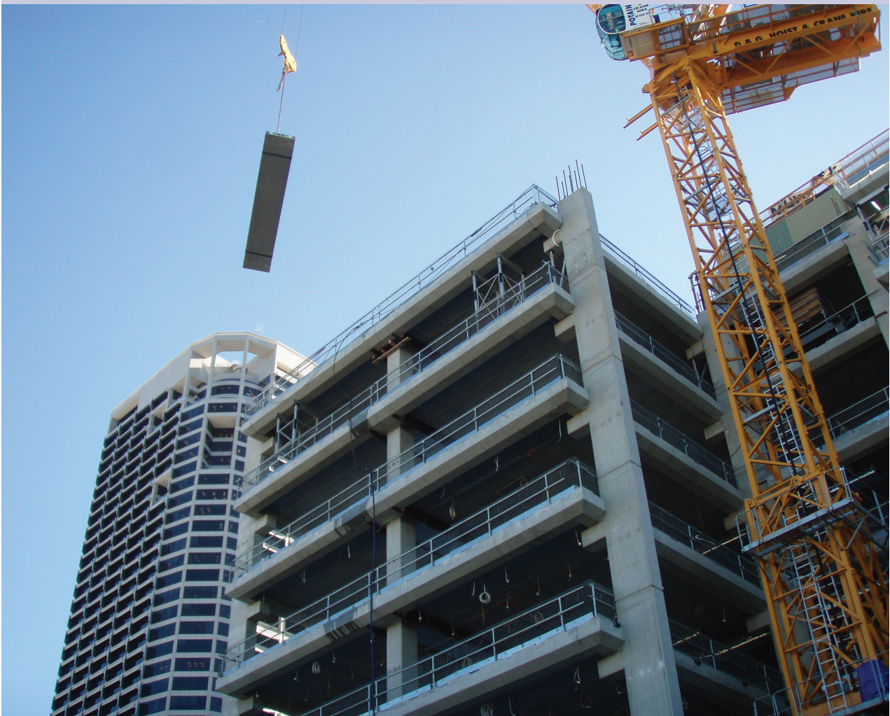
Image 24 – Robust framing to prevent progressive collapse during construction should be considered by the Erection Designer
