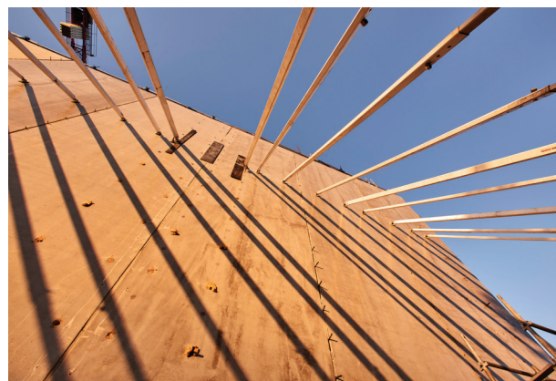
Image 15 – Braces and props are generally proprietary telescopic systems
