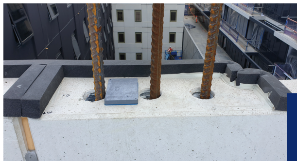
Image 19 – Placement of shims and other joint preparation works
