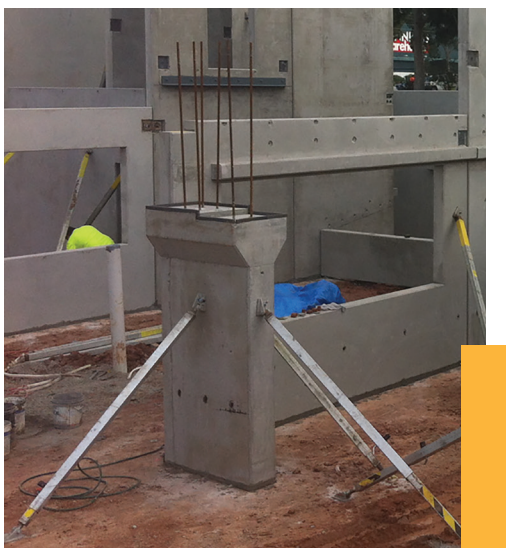
Image 3 – Braced precast columns
