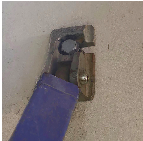
Image 7 – Top brace connection utilising a threaded insert and an M20 class 4.6 bolt
