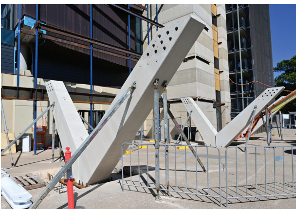
Image 17 – Some elements require both bracing and propping
