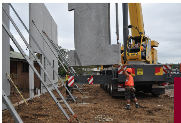
Image 18 – Installation of prefabricated concrete panels
