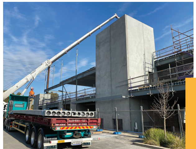
Image 23 – Precast panels forming lift/stair cores may be self-supporting against wind loads once they are interconnected and no longer require temporary bracing
