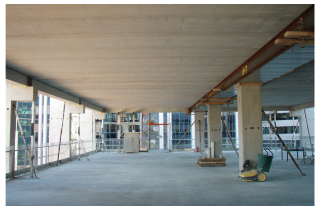
Image 13 – Precast columns with temporary bracing to provide horizontal restraint
