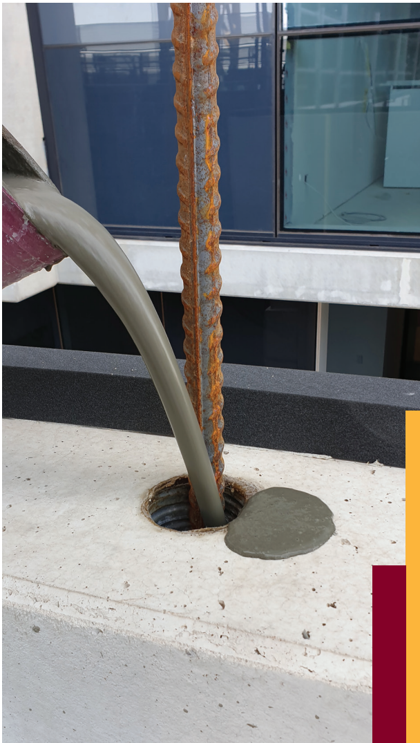
Image 16 – Dowels and starter bars may not provide sufficient lateral restraint until they are grouted and cured
