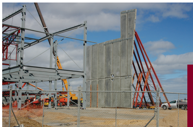
Image 14 - Knee-braces (affording restraint in all directions) may be used to increase compression capacity of telescopic braces
