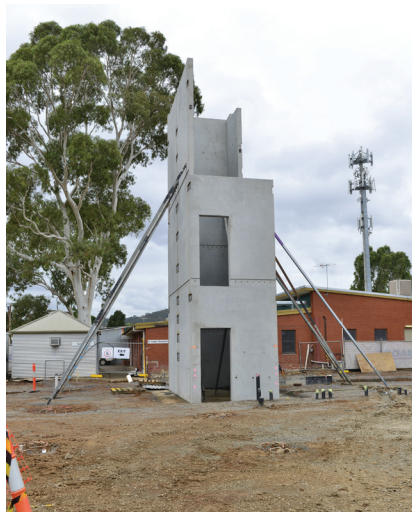
Image 9 – Precast stair shaft braced on opposite sides
