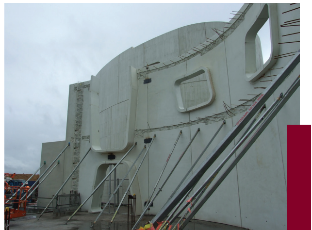
Image 2 – Element bracing design should resist common lateral forces such as wind
