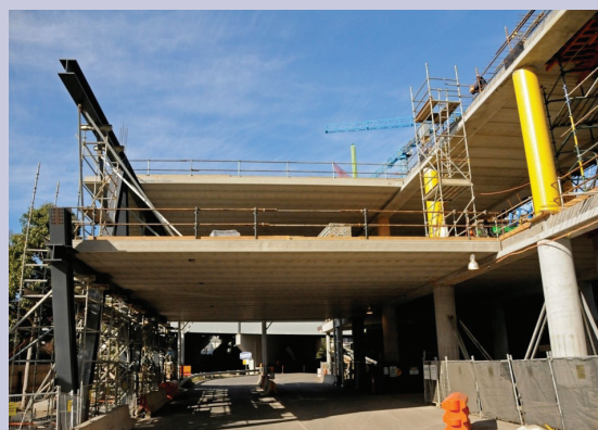
Image 5 – Prefabricated floor units installed on permanent steelwork
