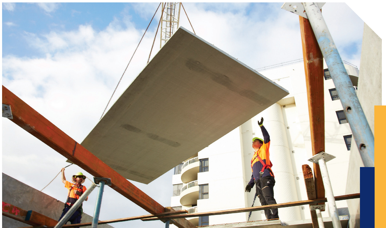
Image 10 – Precast flooring may require propping when the elements are unable to clear span on their own,, especially if a composite topping slab is added
