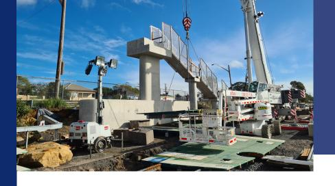
Mr Waeger's company has been involved in the project from the outset, supplying columns, headstocks and stairs for the pedestrian overbridge and also fabricating culverts, L-walls and slabs for the upcoming platform upgrade. In total, when complete, approximately 240 precast items will have been installed.
