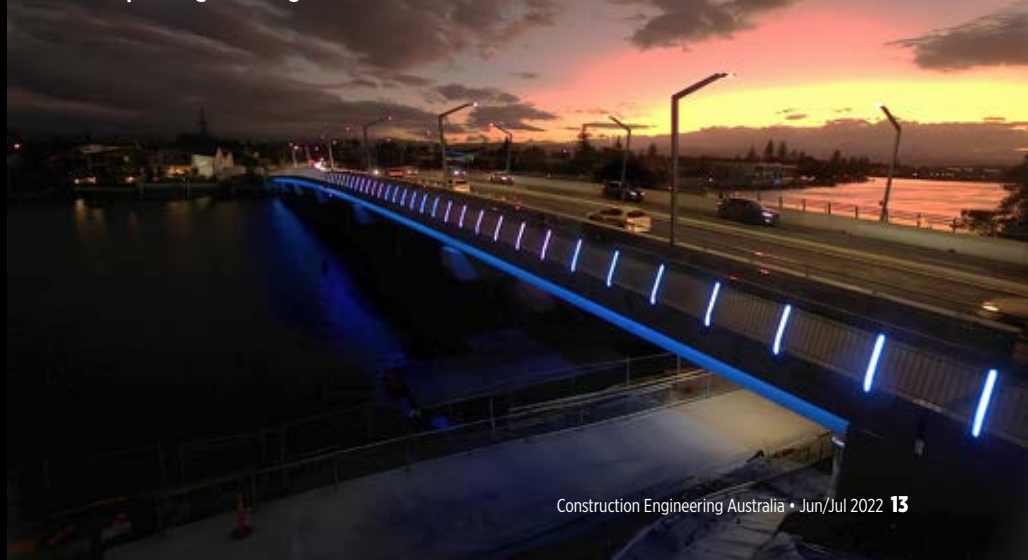
Isle of Capri Bridge at twilight.
