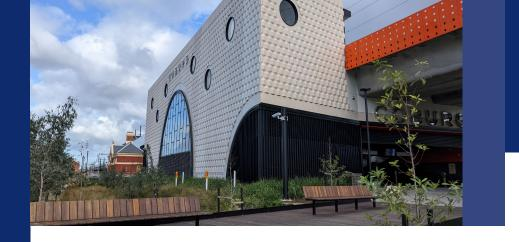
Prefabricated construction methods such as precast concrete greatly reduce the burden of onsite trades and waste, and allow elements to pass thorough a quality control check before their transport to and installation on site. Advanced Precast's implementation of custom form-liner technologies was used to resolve the complex diamond embossed façade panels for the new Coburg station building.
