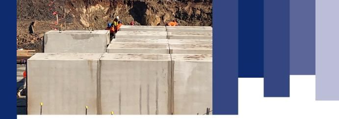
Measuring an enormous  $1.8 \times 1.8 \times 2.4 \text{m}$ , the box culverts were installed on top of the link slabs to form a milti-cell culvert crossing. The link slabs measured  $1.8 \times 1.8 \times$
