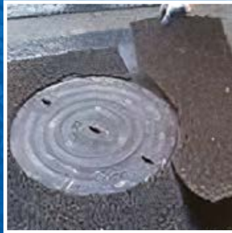
SEALING UTILITY REPAIRS
