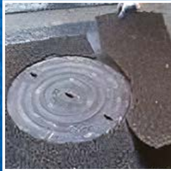
SEALING UTILITY REPAIRS
