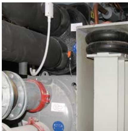
Quiet and hygienic, Marsh Mellow® industrial springs can replace noisy coil springs in manufacturing, food and beverage and other applications where metals pose washdown and breakage issues
