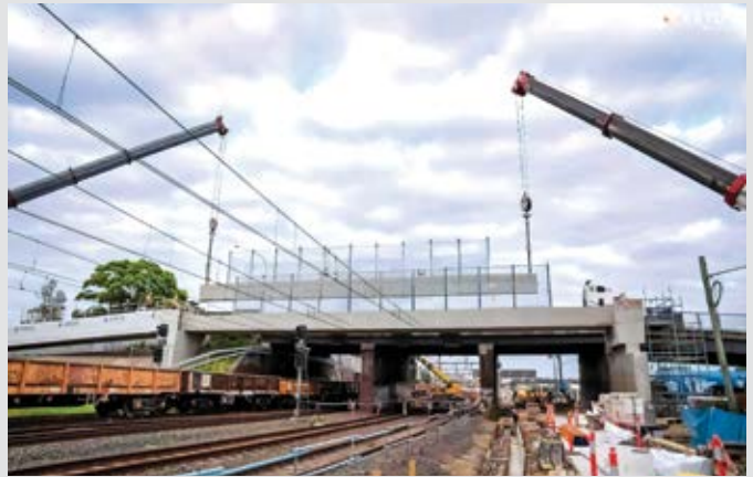
Project: Powering Sydney's Future Location: Sydney, NSW Master Precaster: Waeger Constructions Client: TransGrid Bridge Design / Construction: Certus Projects, Turnball Engineering
