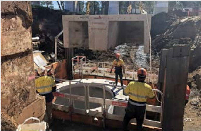
Project: West Dubbo Gross Pollutant Trap Location: West Dubbo, NSW Master Precaster: Rocla Client: Dubbo Regional Council Builder: Whittaker Civil Project Management: Optimal Stormwater
