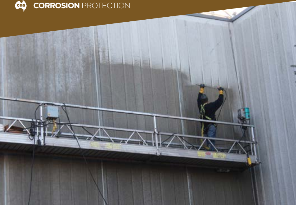
Pictured left: MCI-2018 being spray-applied to the walls of a prefab concrete building. Image courtesy Cortec
