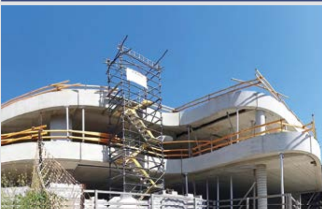
Project: Edzell House Location: Toorak, VIC Master Precaster: Hollow Core Concrete Builder: Surrey Developments
