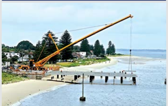
Project: St George Sailing Club Location: Sans Souci, NSW Master Precaster: Alpha Precast Client: St George Sailing Club Developer: Join Construction Architect: Jon Jacka Precast Installation: Total Precast
