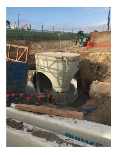
Precast concrete allowed for a reduced congestion of trades on site and a highly efficient installation that took less than one hour from unloading from the delivery trucks.
