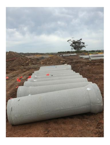
manufactured and supplied. Varying in radii, the pipes were cast vertically and set with an RRJ 2.34m rebate.
