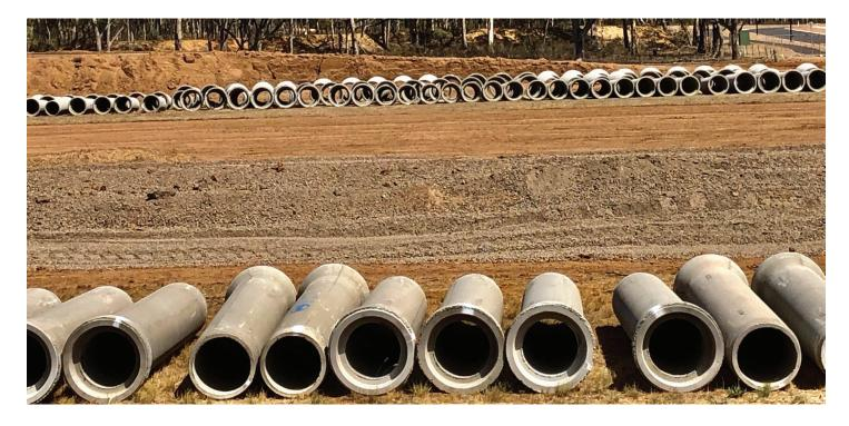
Using precast concrete pipes meant shorter lead times and maximised efficiency on site with fast, safer construction using a minimum of workers. With the units being manufactured in a factory-controlled environment, a high level of dimensional accuracy was easy to achieve, which also minimized challenges along the way.
