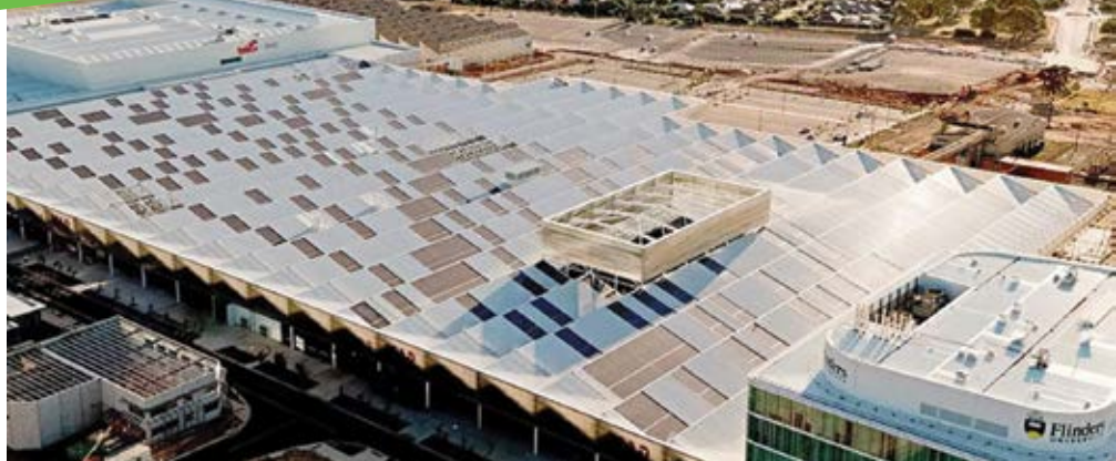
The 7,400 panels are being fitted to the 5-hectare roof of the Tonsley Innovation District in Adelaide south. When complete, the solar array will have a total installed capacity of 2.34MW.
