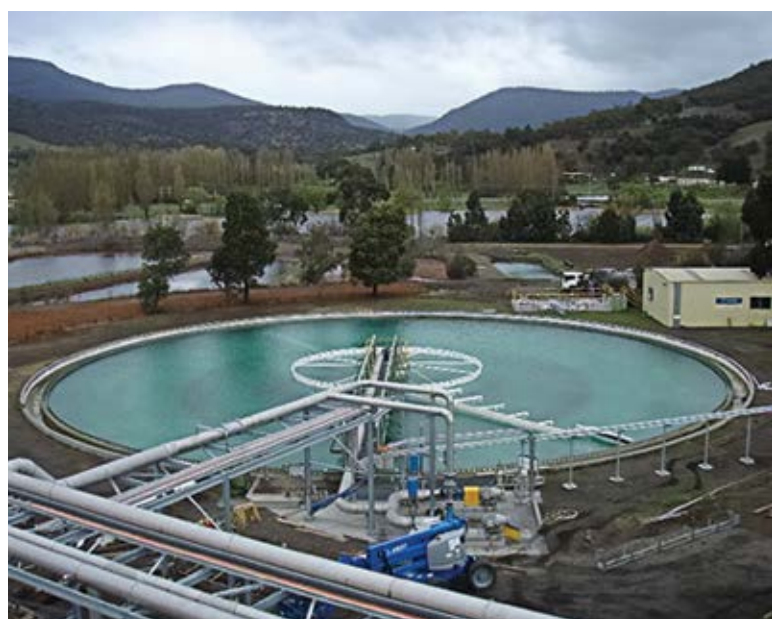
A Smith & Loveless clarifier, installed in Tasmania by CST Wastewater Solutions for the Norske Skog paper mill.
