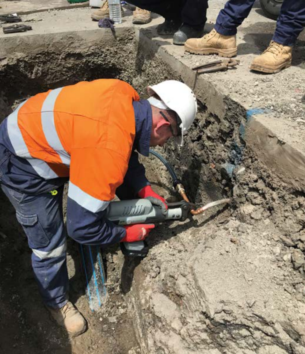
ABOVE: Viega Propress being installed. Image courtesy Viega Australia
