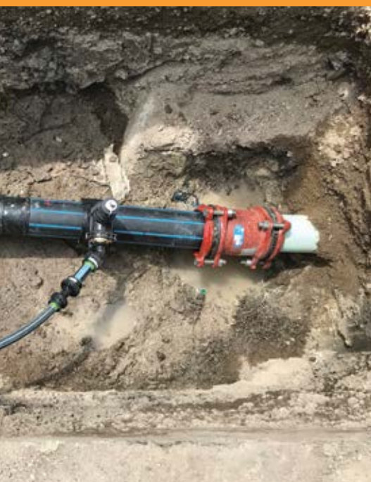
BELOW: Viega Propress and Viega Geopress K being used in the same application. Image courtesy Viega Australia
