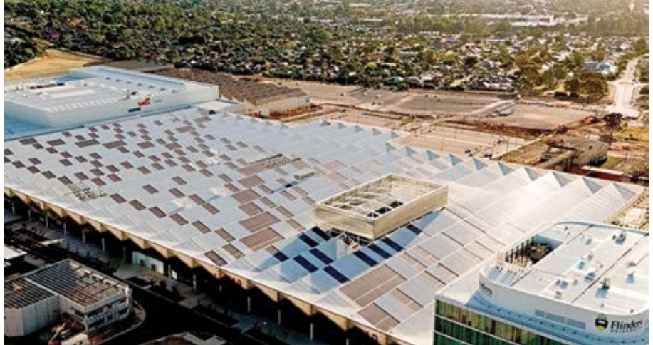
Australian Gas Networks has begun construction of its HyP SA hydrogen production facility at the Tonsley Innovation District in Adelaide.
