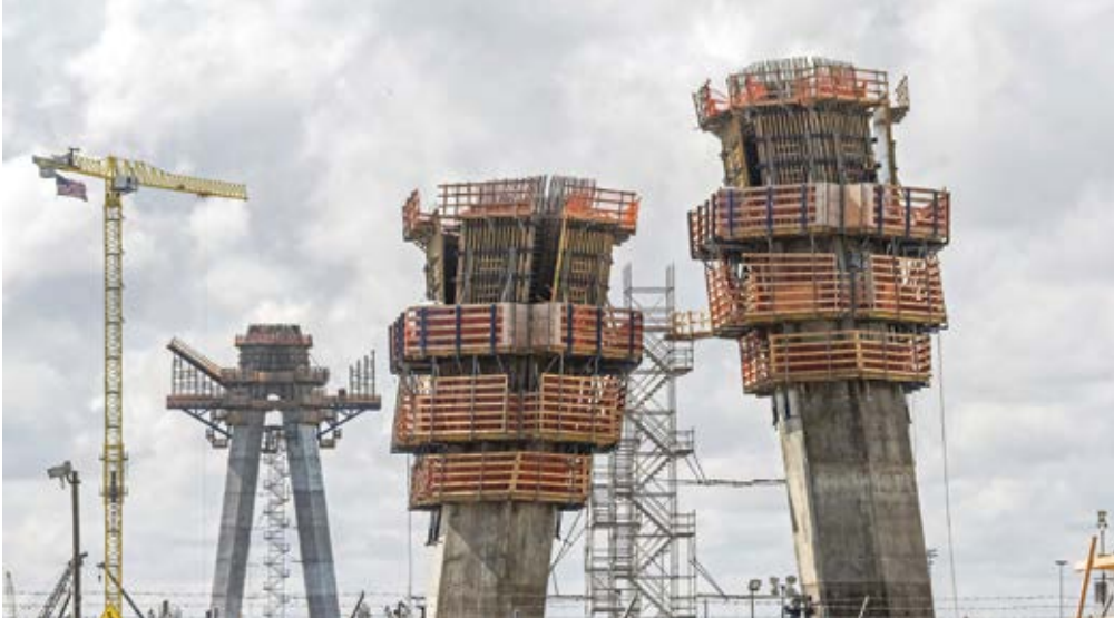
LEFT: The two pylons are 164 metres high, comprising the A-shaped pylon legs and the pylon tower above. Image courtesy Doka ©2020
