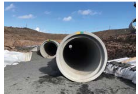
Road and rail infrastructure works are underpinned by drainage systems that incorporate precast elements such as pipes, box culverts and other elements.
