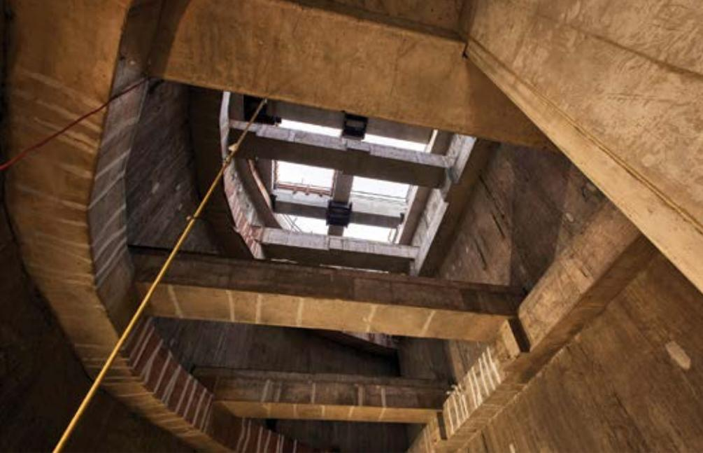
**Above:** The buildings are directly connected to the tunnel via two 35-metre-diameter underground shafts that descend more than 60 metres from ground level.
