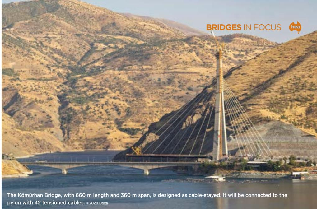
The Kömürhan Bridge, with 660 m length and 360 m span, is designed as cable-stayed. It will be connected to the pylon with 42 tensioned cables. ©2020 Doka
