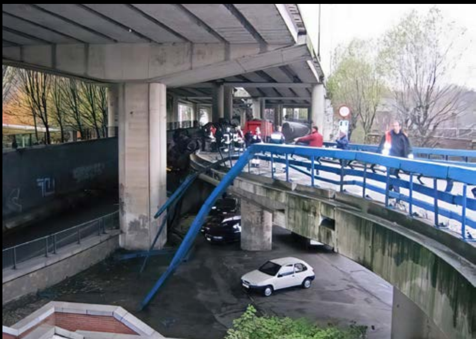
ABOVE: Use of the old style, non-tested, Mailleux parapet design ceased in Belgium following the introduction of the European Standard EN1317.2
