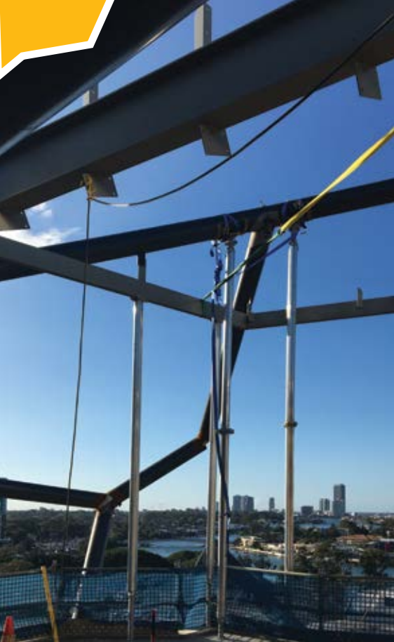
ABOVE: Pop out steelwork in the shape of the voronoi pattern was the most challenging of all steel elements on this project.
