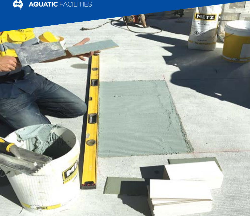
Back buttering a tile on-site prior to laying tiles, using the Tarver method. Note: notches are unidirectional on tile glue surface.
