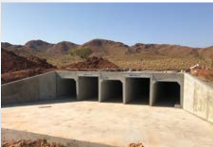
Pipes and culverts were recently supplied to the WA Marble Bar Realignment project (MJB Industries)
