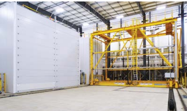
Above: The pallet stacker serves the two racks and stores and retrieves the pallets with the freshly concreted solid wall elements.
