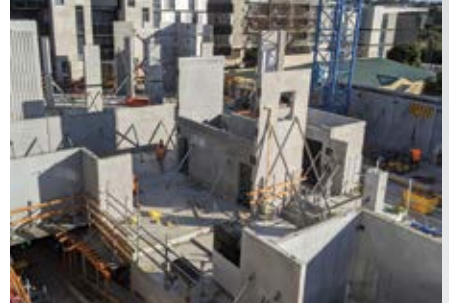
478 panels and 232 columns are being used in Arnold Apartments, Box Hill, VIC (Walker Panels)
