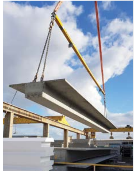
84 super-tees @ 48 tonnes each for the Next DC Tier 4 data centre in Tullamarine, VIC (Hollow Core Concrete)
