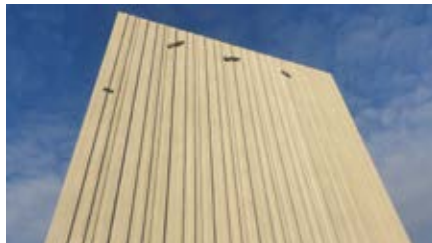
148 panels, 13.5 metres high using formliners were manufactured for UTAS Cradle Coast Campus, TAS (Duggans Precast)
