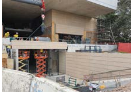
Acid-washed panels for the University of Sydney's Chau Chak Wing Museum, NSW (Precast Concrete Products)
