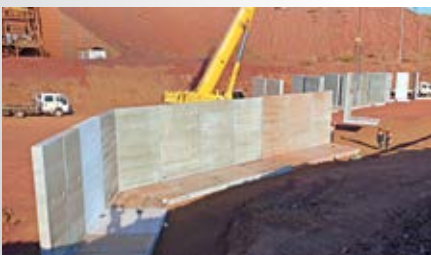
Precast arch tunnels and L-shaped retaining walls for the Pilbara's Mesa A Grade Separation, WA (Reinforced Earth Co)
