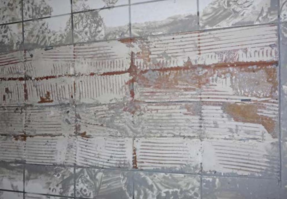
Left: Typical view of failed tiles with trowel grooves of variable direction, many gaps for water migration, glue fragmenting and insufficient adhesive coverage.
