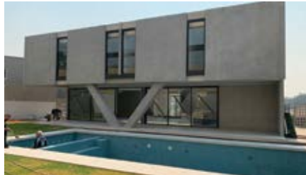
105 panels were supplied for this precast home at Connells Point, NSW (Alpha Precast, erected by Total Precast)
