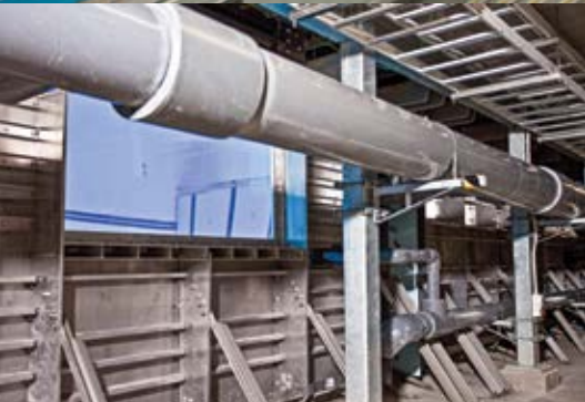
From above, the pools at the Marion Aquatic Centre in suburban Adelaide would appear to the untrained eye, to be no different to any other large competition pool. The view from below ground (pictured left) shows the pool's engineered stainless steel panels and supports.
