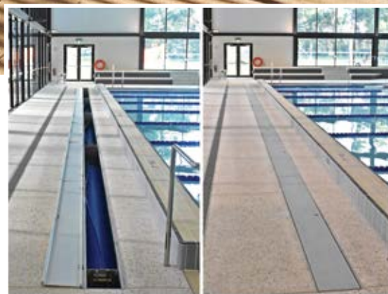
Now you see it – now you don't. This built-in pool cover system makes the most of valuable space by storing the pool cover under the pool deck when it's not in use.
