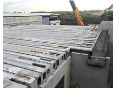
Melbourne-based precaster Hollow Core Concrete manufactured and installed over 8,000m 2 of their signature hollowcore prestressed floor planks for the project.
