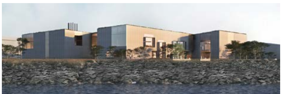
Top: National Precast Master Precaster Duggans Precast supplied a total of 148 precast concrete panels for the project. Above: The precisely formed panels cover a total surface area of 2030m 2 . Image courtesy University of Tasmania
