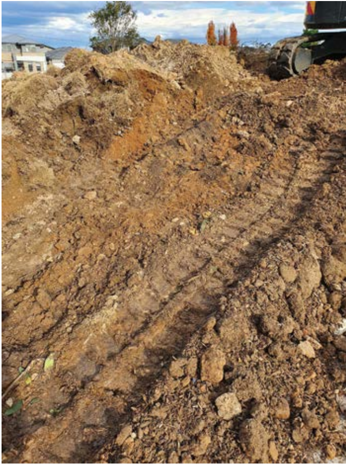
Figure 2. Heavy compaction results from traffic over stockpiles
