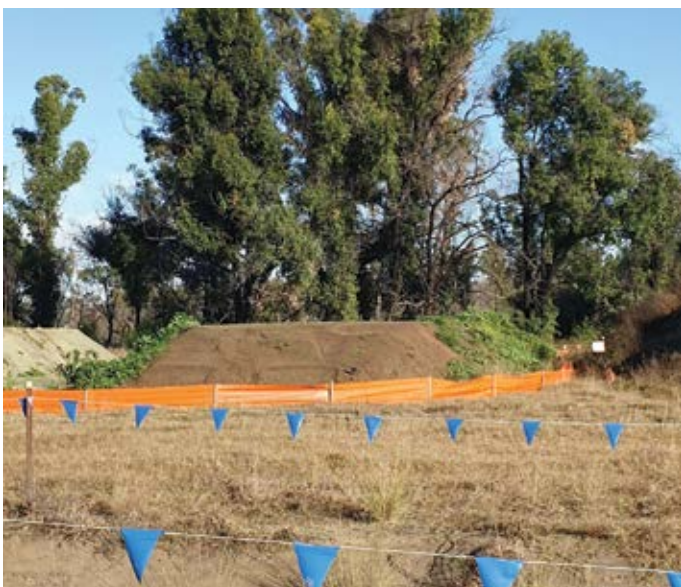
Figure 3. Flat top to reduce erosion and erosion control to minimise soil loss. Traffic is also excluded.
