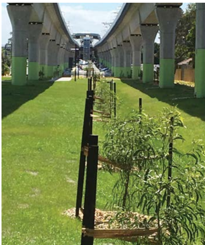
Figure 1. Completed section of the Caulfield to Dandenong Level Crossing Project
