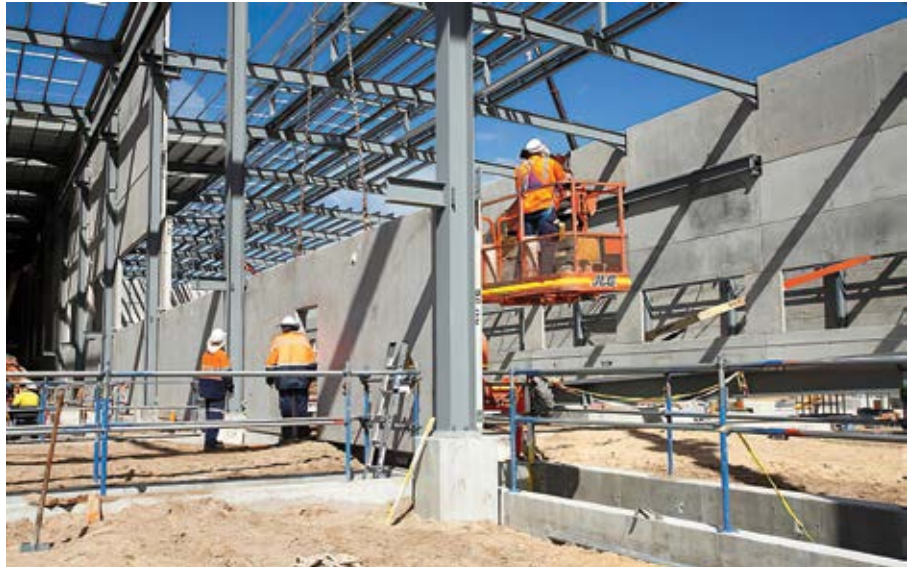
Being manufactured off-site, precast offers safer and more efficient construction, and its use should be encouraged during the Covid-19 pandemic.
