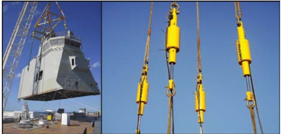
Above: (LEFT) Enerpac SyncHoist technology has also been employed in Australian naval construction for precision positioning of major components. (RIGHT) Enerpac SyncHoist utilises four lifting and control points suspended from one crane.
