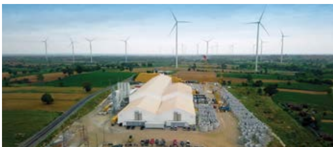
Mobile plants enable flexible, just-in-time production. Photo: Courtesy Firmengruppe Max Bögl ©2020
