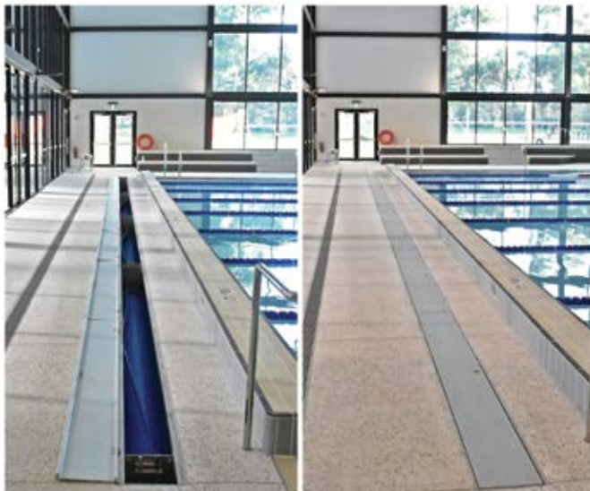
This state-of-the-art built-in pool cover system makes storage easy - storing the pool cover under the pool deck when it's not in use.
