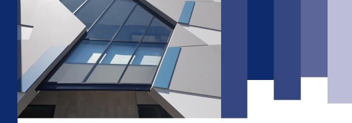
The unique geometry and 3D nature of the shopping centre's façade posed challenges during installation. Accurate alignment was critical to achieve the desired design result. Overcoming the alignment difficulties, which arose from a combination of recessed and protruding panels, hinged on an experienced precast installer. Asurco was up to the task, and the resulting facade is a testament to the company's experience.
