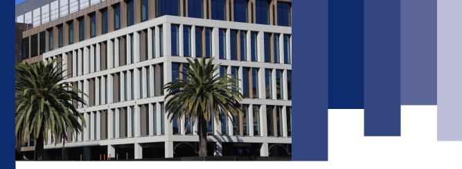
of the project, accommodate site requirements and fast-track the project's construction programme. With construction of the building running from April 2018 to October 2018, Delta manufactured precast concrete flooring, structural columns, structural beams and facia panels for the project.
