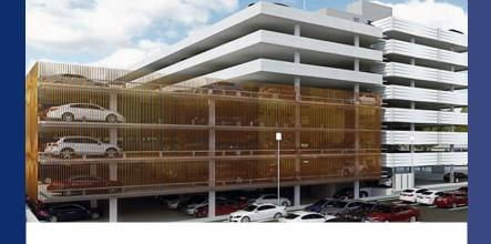
All elements were manufactured with 40MPa off-white concrete mix, with 6% titanium dioxide colour oxide. The patterned panels have a 30mm vertical relief, while the plain panels have adopted a Class 2 off-form finish
