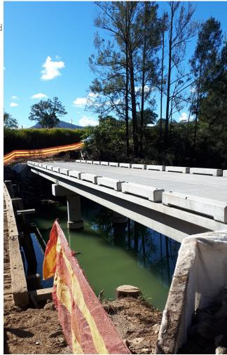
The Bridge Replacement Program is part of the Council's 10 Year Works Program 2017 – 2027 and includes the replacement of 94 timber bridges. Timber bridges constituted 73% of the Council's bridge assets before the program began, with 28% of those being identified in poor condition. It is projected that over the next 25 years all timber bridges will have been replaced with concrete/composite structures or reinforced concrete box culverts.
