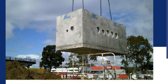
Despite the geographical distance of just more than 150 kilometres between MJB'S factory and the worksite, using precast significantly reduced on-site construction times. The total amount of time saved for the client was approximately five weeks—one week per tank.
