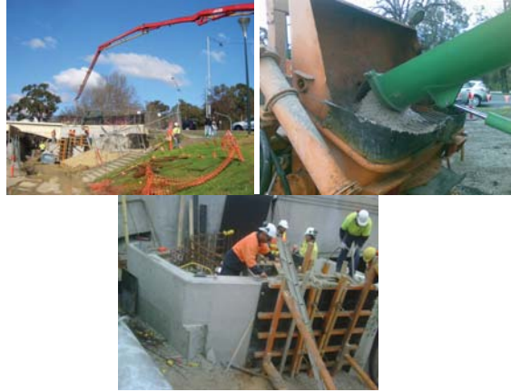
Fig. 4. Construction of geopolymer concrete retaining walls using conventional techniques
