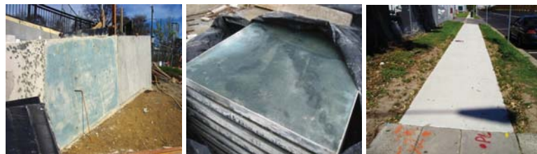
Fig. 2. Geopolymer concrete, retaining wall (L), footway panels (C) and footpath (R)
