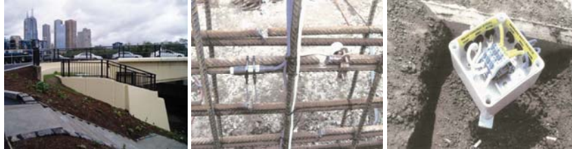
Fig. 6. Finished painted wall and installed reference electrodes
