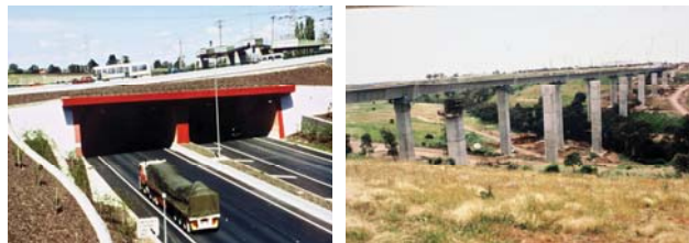
Fig. 1. Jacana Tunnel and Whitten Bridge (Western Ring Road) constructed with significant amounts of SCMs
