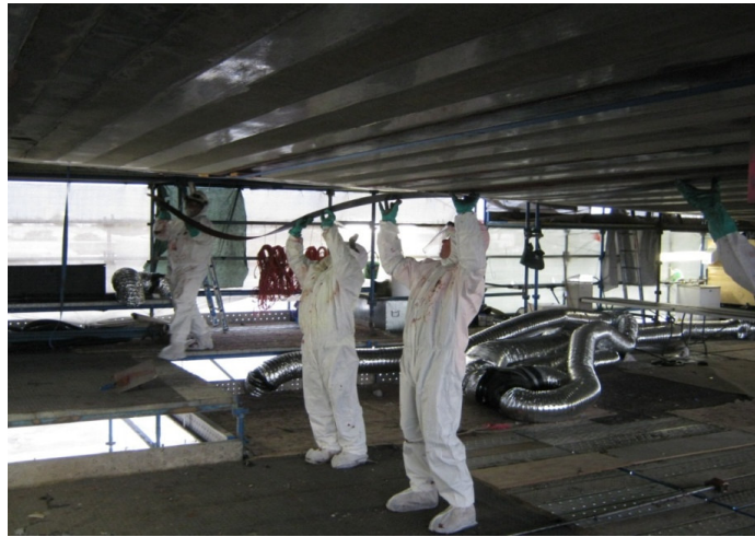
Fig. 12. Installation of 14m long carbon fibre laminate
