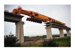
New technology in China is making bridge girder installation a breeze. The SLJ900/32 made by Beijing Wowjoint Machinery Company is a machine that replaces the need for a crane. Watch SLJ900/32 in action in this great timelapse video.
