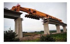
New technology in China is making bridge girder installation a breeze. The SLJ900/32 made by Beijing Wowjoint Machinery Company is a machine that replaces the need for a crane. <u>Watch SLJ900/32 in</u> <u>action in this great timelapse video.</u>
