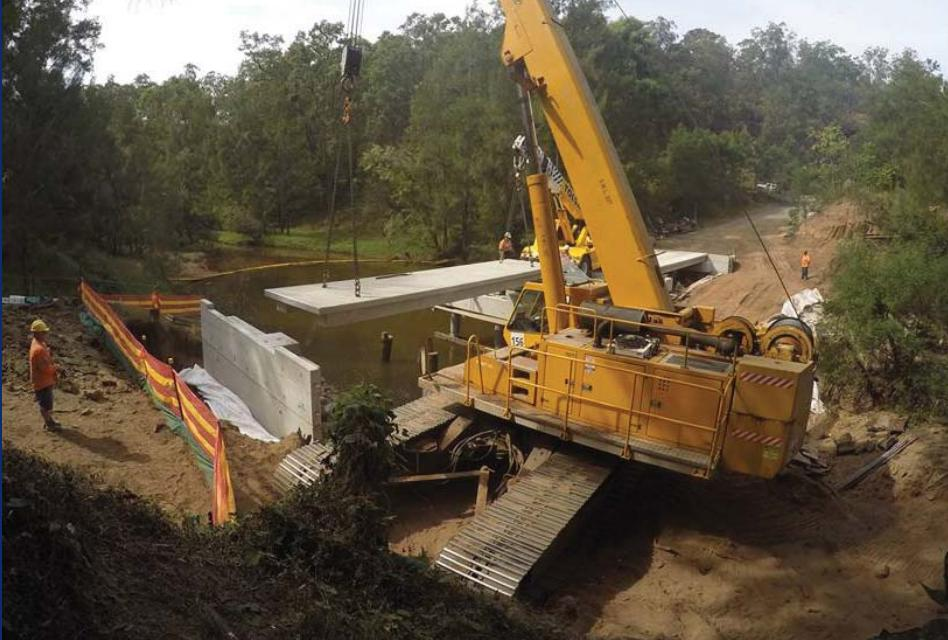
Waeger manufactured all the components for the new 30 metre long and 4.5 metre wide single lane bridge. That included precast abutments, head stocks and also Waeger deck bridging modules.
